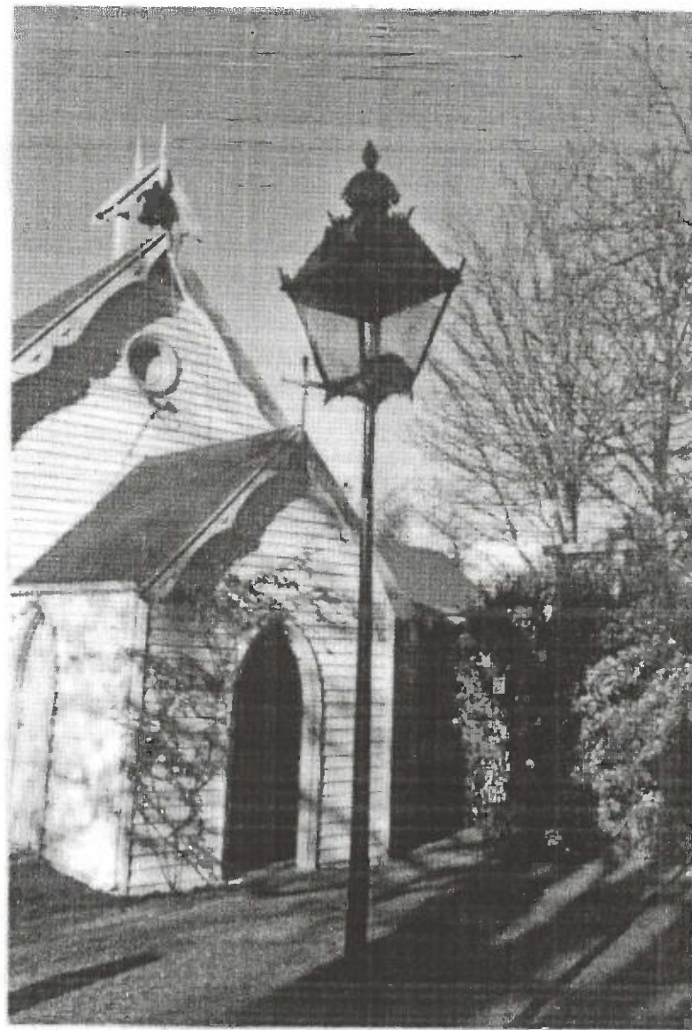
Saint Paul's Anglican Church, Arrowtown By Rupert Iles, September 2000
